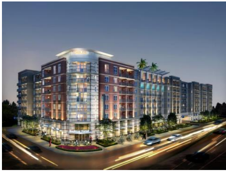
Gables Tanglewood, Houston, Texas. In-progress
