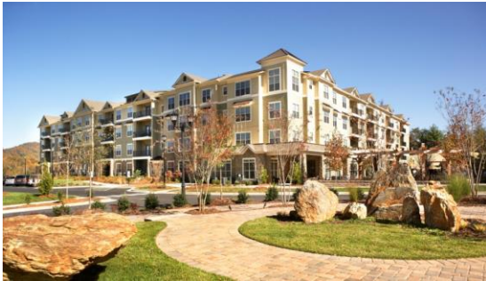
Verde Vista, Asheville, North Carolina > 252 units; 280,000 total SF > 0.124% Increased cost (as a % of total) or $79/unit for NGBS Silver > 0.62% or $396/unit for Energy Star certification
