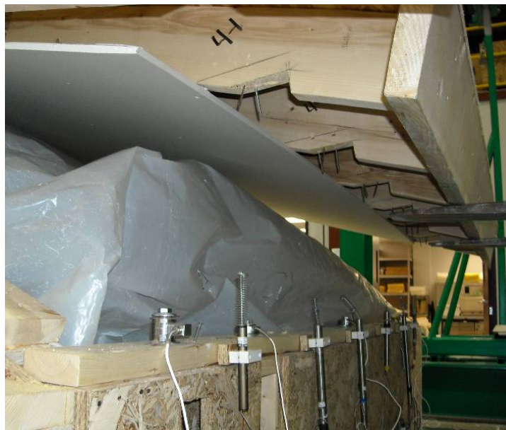
Figure 11 – Specimen after failure
