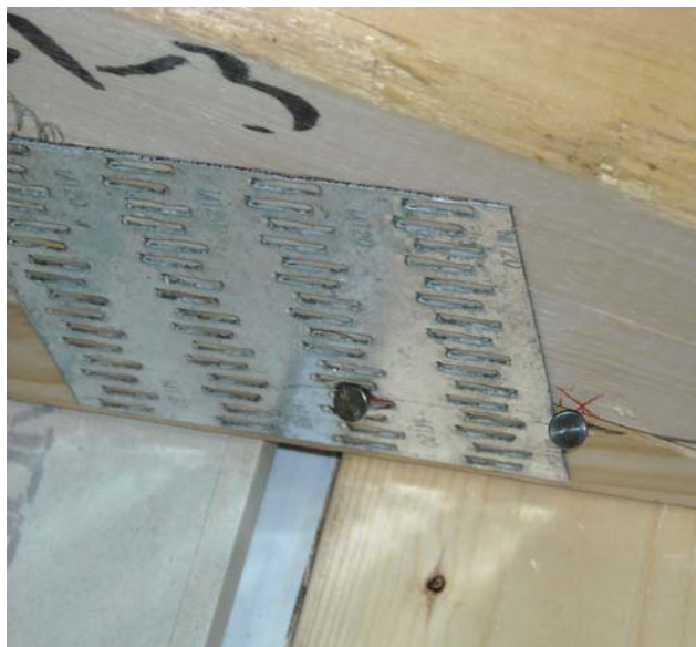
Figure 19 – Installation of one nail through the truss plate and one nail adjacent to the truss plate
