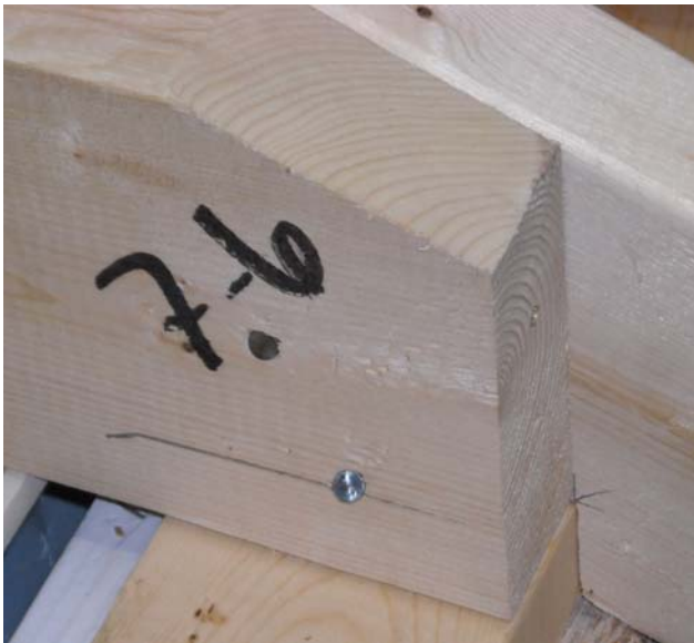
Figure 8 – Installation of toe-nails
