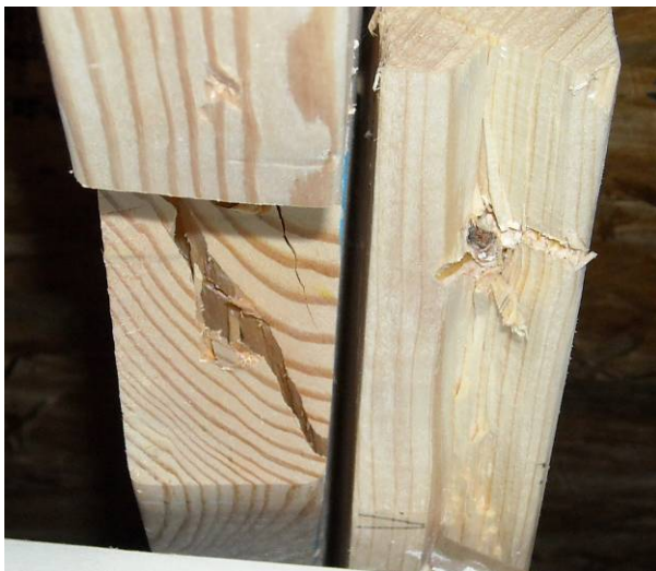
Figure 17 – Pull-through failure of all ring-shank nails
