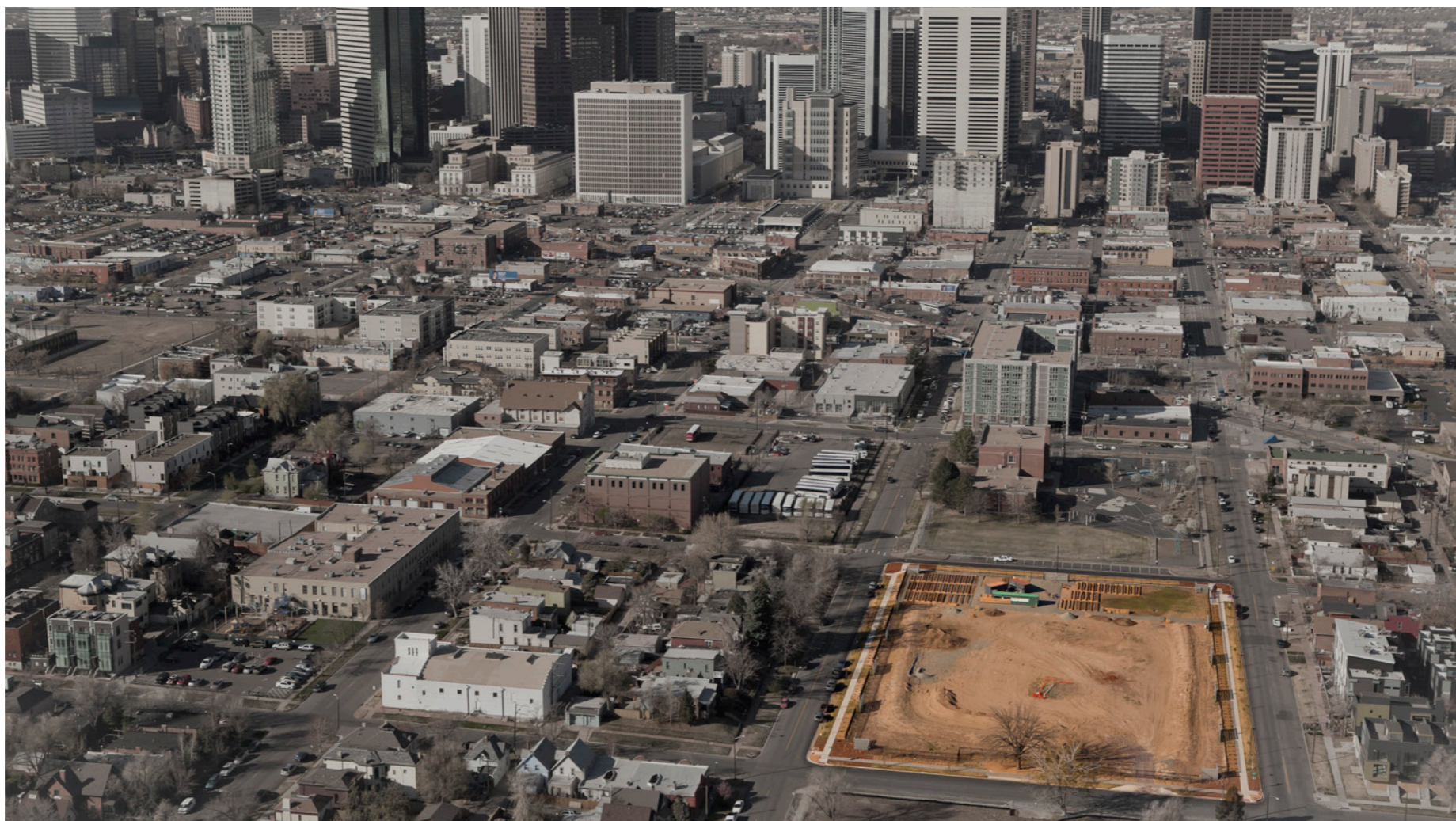
Aerial View to South West
